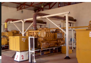
ТОО «TOLKYNNEFTEGAZ» POWER PLANT BASED ON CATERPILLAR GAS GENERATOR SETS
