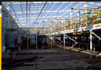
ТОО «TOLKYNNEFTEGAZ» POWER PLANT BASED ON CATERPILLAR GAS GENERATOR SETS
